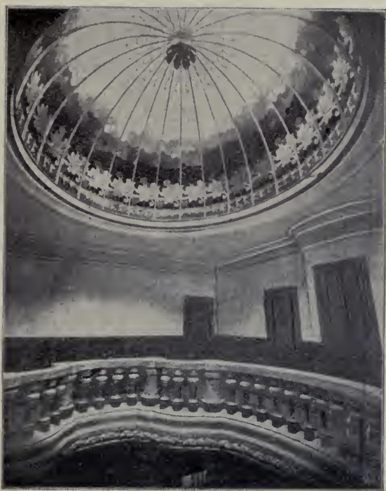
No. 4 AVENUE D' JENA. (Dome over Staircase.)
